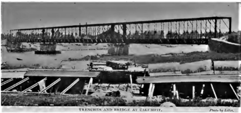
TRENCHES AND BRIDGE AT CALUMBIT.
