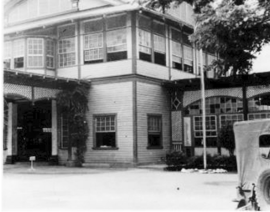
Administration building of the former Bamban Sugar Central (Central Luzon Milling Company) used as cell and torture chamber for suspected local guerrillas, circa 1945. From the National Archives and Records Administration (NARA).
