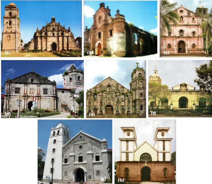
Figure 1. (a) Church of San Agustin, Paoay, Ilocos Norte; (b) Church of Our Lady of the Assumption, Santa Maria, Ilocos Sur; (c) Church of Pope St. Gregory the Great, Majayjay, Laguna; (d) Parish Church of the Holy Cross, Maribojoc, Bohol; (e) Church of Our Lady of the Gate, Daraga, Albay; (f) Parish Church of St. John the Baptist, Jimenez, Misamis Occidental; (g) Church of the Assumption of Our Lady, Maragondon, Cavite; (h) Church of the Immaculate Conception, Jasaan, Misamis Oriental
