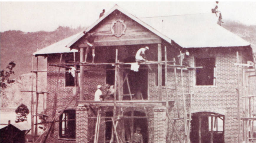
Figure 7. Home Economics Building being built with local materials ( Annual Report 1927 )
