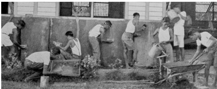
Figure 9. Grade VII pupils constructing the school's shop building ( Annual Report 1932 )
