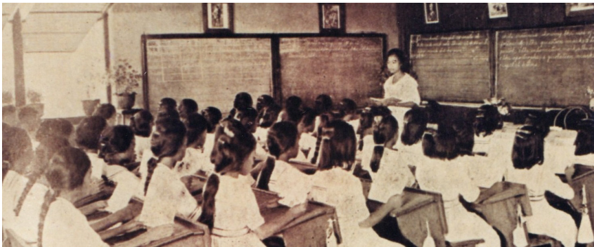
Figure 3. Classrooms with swing-out capiz windows to let in fresh air ( Annual Report 1922 )
